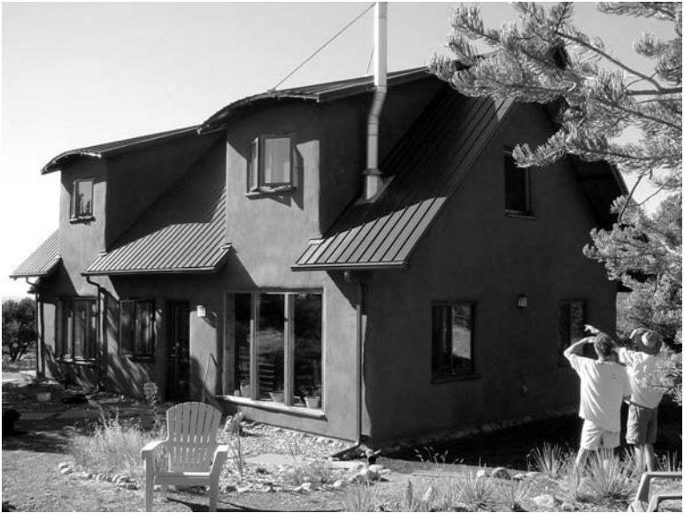
Figure 6.8 A straw-bale house built in a mainstream style by Paul Koppana, Crestone, Colorado
