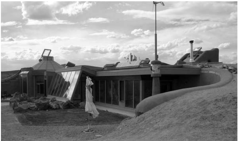
Figure 6.6 An autonomous Earthship, showing south-facing greenhouse front and earth-banked rear, Taos, New Mexico
