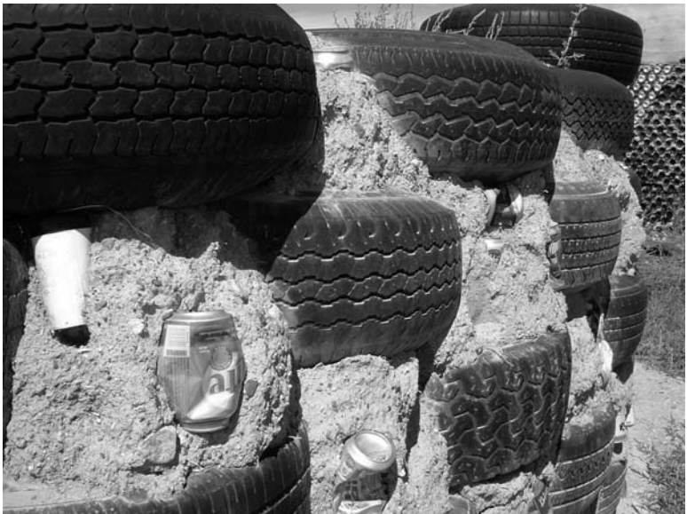
Figure 6.7 Earthship walls made of tyres, earth, bottles and cans
